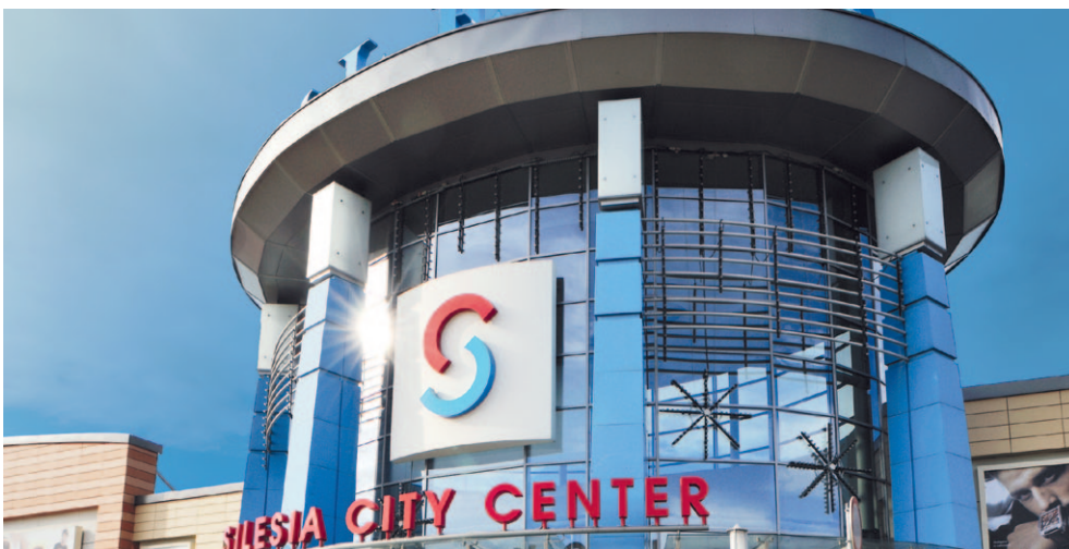
Silesia City Center, Katowice, PL
