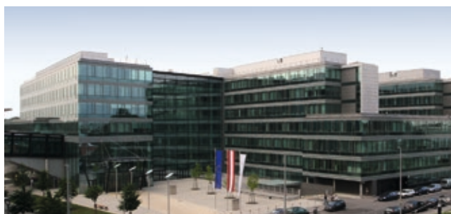
Office Campus Gasometer | Vienna | AT
